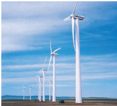
One-hundred tonnes of steel are used for affordability and strength in a 60 metre wind turbine tower.
